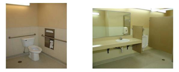
The faucets use handles that must be pushed and held down to keep water running. These can be difficult for some individuals with a mobility disability to use, so the team suggested that handles be exchanged with larger flipper handles.
