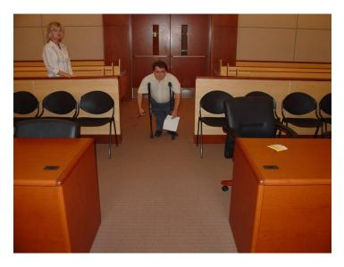
The witness box had an easy slope, with rails, at approximately 36 inches, making for a fully accessible witness box. The witness chair was on casters and therefore could be removed to accommodate a witness using a wheelchair.
