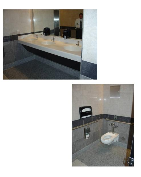
The sinks used a wood cover over the pipes, instead of pipe wraps, sloping down and away from the sink at a 45 degree angle. While this wood cover was common in courthouses in Maricopa County, the barrier makes it difficult for a person using a wheelchair to pull close to the sink. Otherwise, the sink is at an appropriate height.
