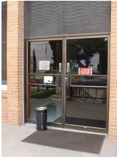
The accessible entrance could be a lighter tension, but was slow-closing, which is helpful for persons with mobility challenges. Light tension doors can be used at entrances, without the door being subject to wind or air pressure pulling it open.
