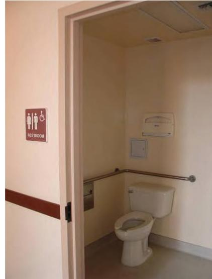
The third floor has a unisex bathroom, but with Braille description. Braille identified all of the bathrooms in the building. That bathroom was fully accessible, including wheelchair entry and exit space, heat wraps on the sink pipes, and a soap dispenser to the sidewall, making it easier to reach.
