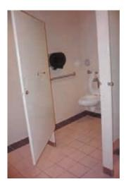
Also in the restrooms, the towel and soap dispensers should be lowered. The faucets in these bathrooms have a "push type" lever. In other words, to turn on the water, the user must push down on the handle. The faucet runs for several seconds, and then shuts off. This is a great way to conserve water, but these types of faucets are difficult to operate. We recommend at least one sink in every bathroom have wing handles which are easier to operate.
