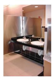
The sinks are excellent, with pipe wraps, but with the faucet controls and the soap dispenser requiring an extended reach, for a person using a wheelchair. The faucet has a push valve at the top of the faucet head, which is quite usable. The length of the sink was over ten feet, leaving considerable room for a person with mobility impairments to operate at the sink.
